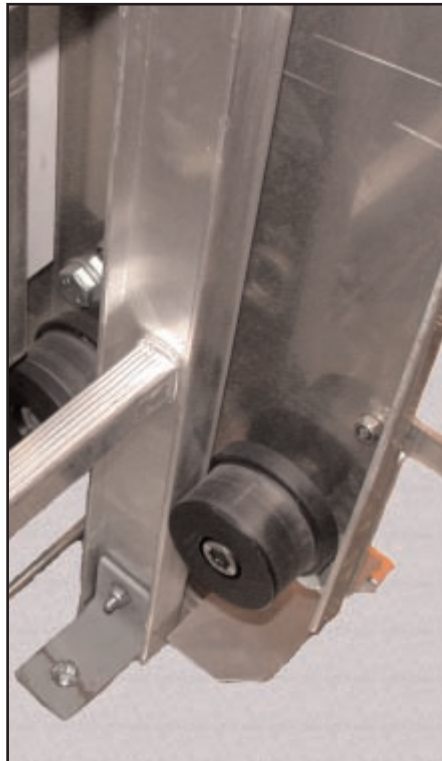
Base of emergency ladder/guide rails showing securement to concrete landing.
