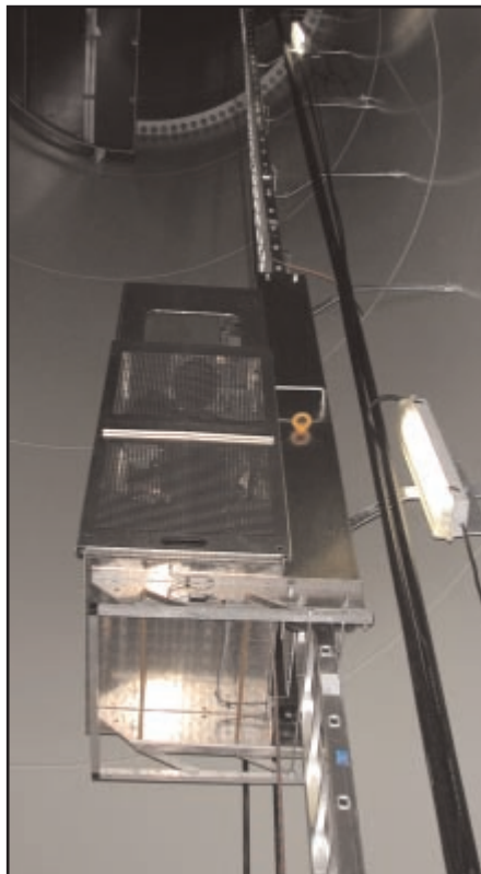
Worm's eye view of wind turbine tower hoist showing how support frame and undercarriage are secured to metal ladder.
